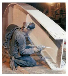
polyurethane topcoat. The aluminium coating should guarantee a protective, maintenance free surface well in excess of 20 years, in a difficult access environment, such as over a motorway, railway or river.
